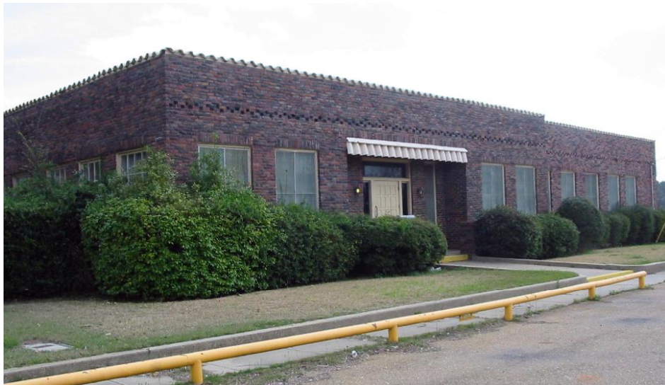
International Paper Co. BagPak Office Building 2004
